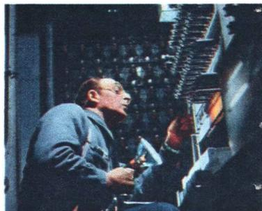
Nat checks complicated electrical relays in sign's control hut. If something breaks down he will keep lights going until day crew makes lasting repairs.
